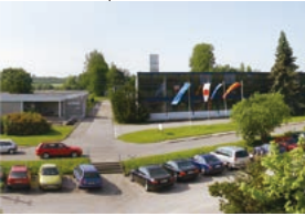
Sumitomo(SHI) Cyclo Drive Germany GmbH (Munich, Germany)
